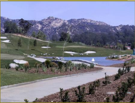
More recent stormwater management facilities include Reidy Creek Golf Municipal Course designed to improve water quality, control flooding, and provide open space and recreation (above)
