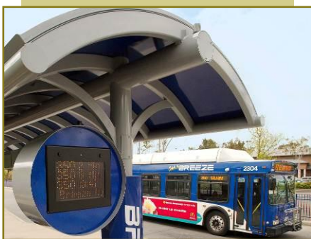
Features of the Escondido's Rapid Bus service include specially designed shade structures, solar powered LED lighting, seating, and electronic displays announcing BRT arrival times (above and right)
