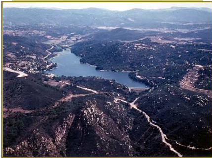
Water diverted from the San Luis Rey River gravity flows through a 14-mile canal excavated by hand in the 1890s through the Paradise Mountains to Lake Wohlford (above).
