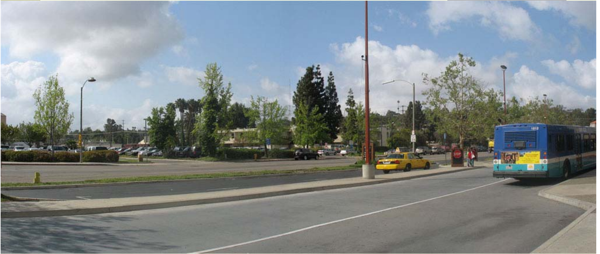
TRANSIT CENTER/POLICE STATION REDEVELOPMENT - ESCONDIDO
